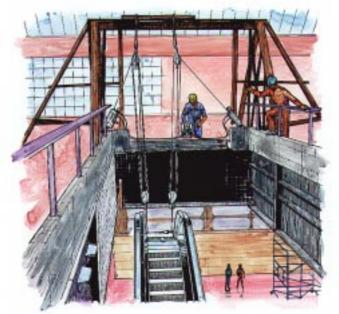
Fig. 27 - Installation of mechanical escalator (TU-16H)
